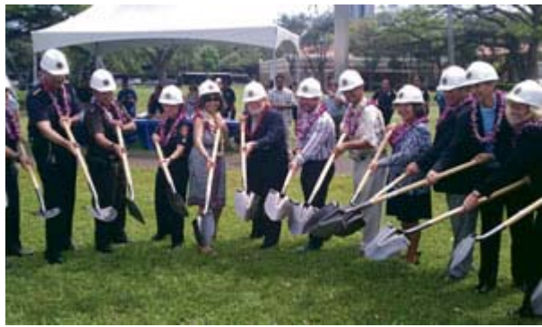
Breaking ground for the fallen officers memorial last Monday. Ron Mizutani photo
